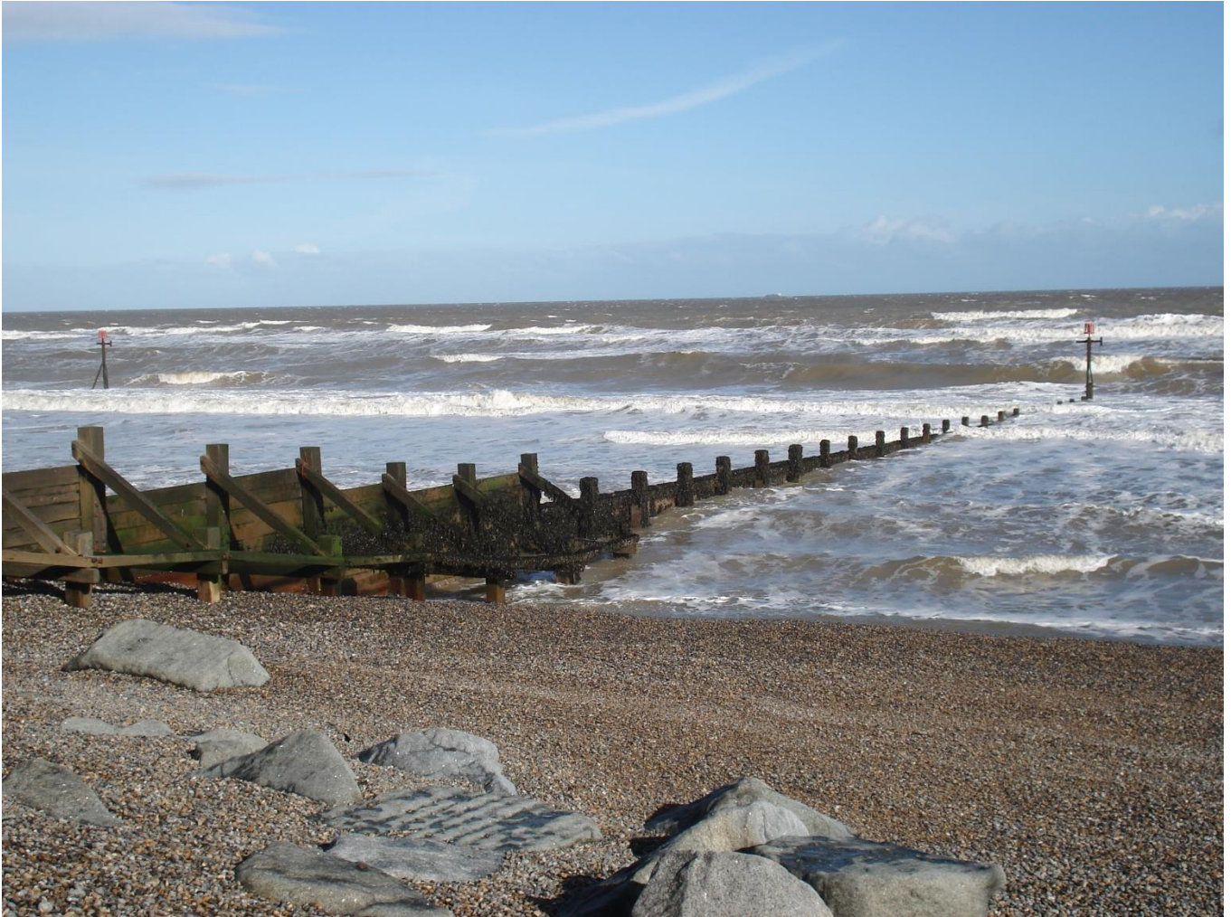
Photograph of groyne at Sheringham
