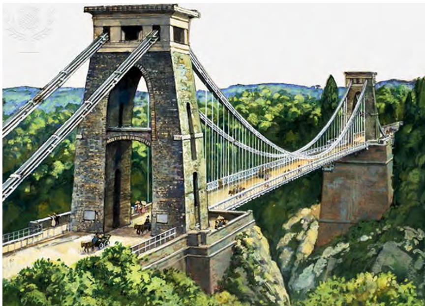
Clifton Suspension Bridge
