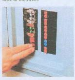
Electricity. Flip off breakers if you find fallen or loose wires or appliance damage, or if you smell burning insulation.
