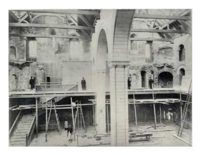
Modern arches, designed to look Norman like the Keep, were inserted to hold up the new roof, and a wooden walkway inserted around the edge
