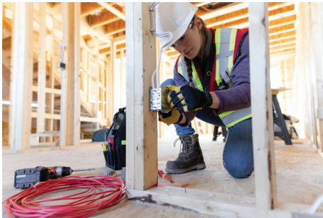
Electrician Installs, inspects and tests electrical equipment
