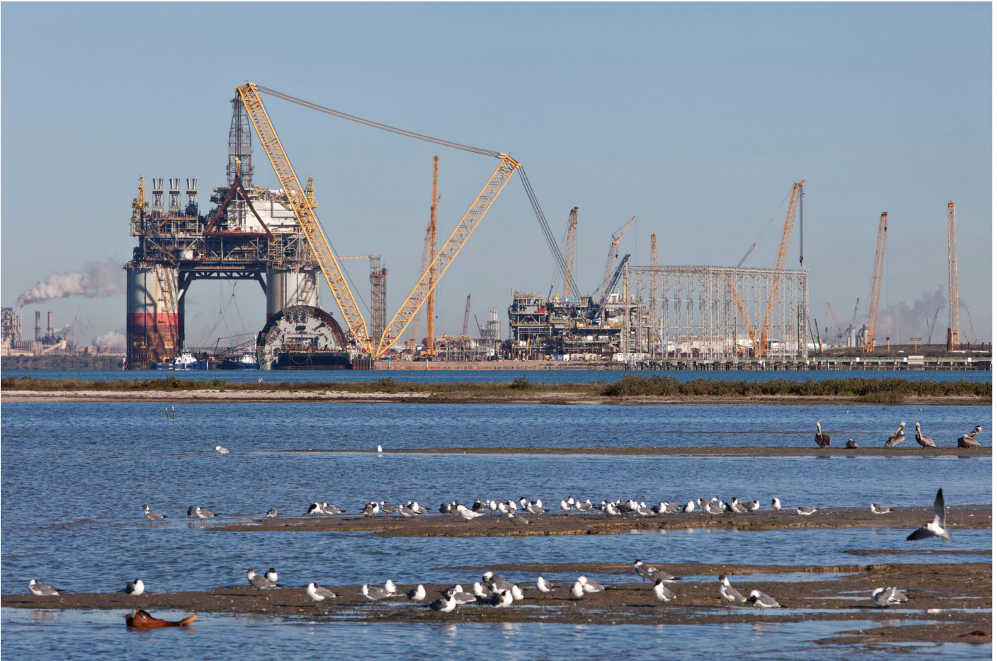
Fig. 8 – Deepwater oil rig under construction, Ingleside Bay, Gulf of Mexico, USA
