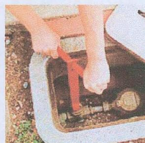
Water. If your water lines are broken, shut off water at the main valve at the street.
