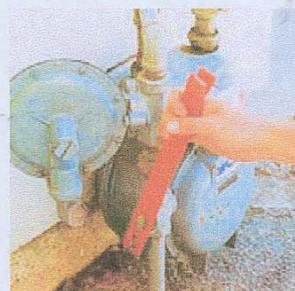
Gas. Shut off gas at the meter only if you suspect a leak.
